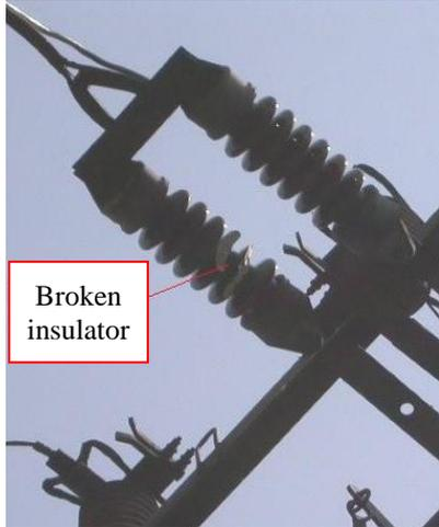
Fig.11. Broken insulator detected by temporary faults
